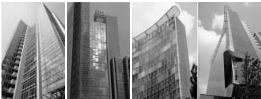
Figure 7.7 The two pictures to the left show the south façade of the debis Haus (1997) in Berlin, Germany. The outer skin of the double façades is made of glass lamellas that can be opened ( far left ) or closed ( left ). The two pictures to the right show the west and south façade respectively of the GSW Headquarters (1998) in Berlin, Germany. The picture to the right illustrates Louisa Hutton’s analogy to a fur in her description of the façade’s appearance. The picture to the far right illustrates the changing effect of glass relative to the angle the façade is viewed from. The appearance of a double façade can also change dramatically with changing daylight conditions. The picture shows furthermore the accentuation of the double facades in the south façade as a narrow vertical stripe.
