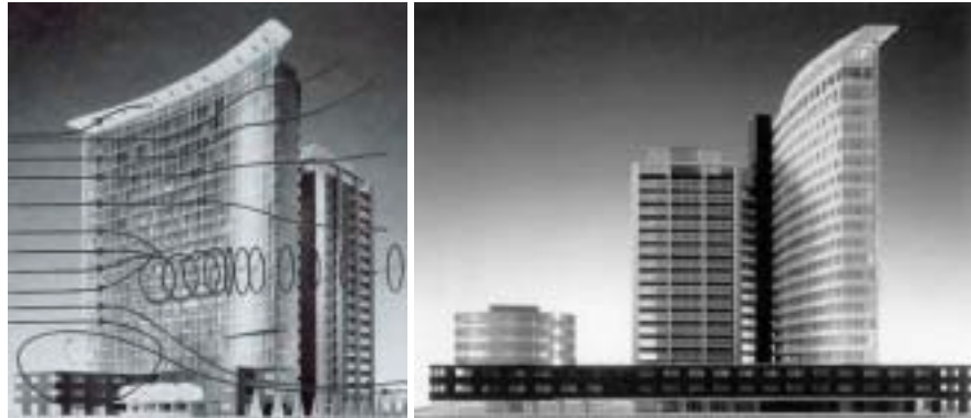
Figure 4.18 The new high-rise building serves as a wind shelter for the existing tower, protecting it from the prevailing westerly winds ( left ). The new high-rise building also shades the existing tower from the afternoon sun ( right ).
