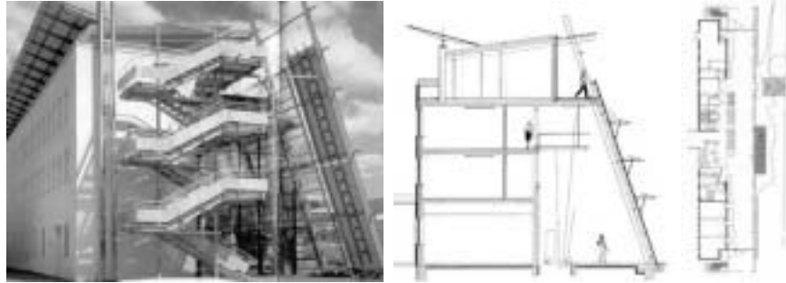
Figure 22 A tilted south façade clad with photovoltaic cells distinguishes the Solar-Fabrik ( left ). Drawing of the section ( middle ) and drawing of the plan ( right ).
