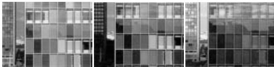
Figure 7.8 The double façade of the GSW Headquarters comprises three layers; a double-glazed aluminium curtain wall, solar shading devices manifested in perforated and lacquered aluminium shutters, and a single-glazed outer skin. The pictures show the changing reflection characteristics of the façade for three daylight conditions. The degree of reflection increases from left to right, while the perception of depth in the façade decreases, as one apprehends only the outer skin. The expression of the façade appears very three-dimensional for some light conditions, the result resembling a holographic image.
