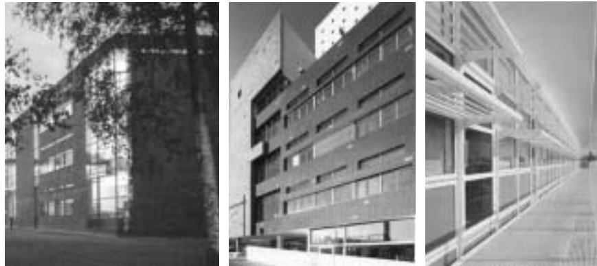
Figure 7.15 Like the south façade of the office wing in the B&O Headquarters, the façades of both the Pihl & Søn Headquarters building ( left ) and the Enschede Tax Office building ( middle ) are characterised by the narrow window bands located above the panorama windows. The narrow windows enhance utilisation of daylight in the interior and provide ventilation openings. (Vents are located right above the daylight windows in the Tax Office). Their size/proportion and location right under the ceiling make them favourable for night-cooling without the risk of burglary. Four bands of windows make up the glass façade of IONICA Headquarters ( right ), where the upper band can be opened and used as ventilation inlets. The south façade of the building is characterised by the fixed solar shading devices.
