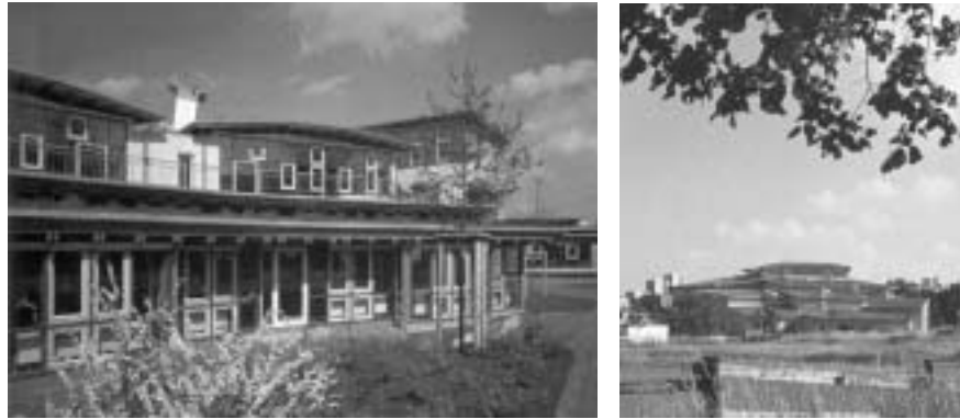
Figure 7.33 A single ventilation chimney with a light, bird-like, shape thrones over the Evangelische Gesamtschule in Gelsenkirchen, Germany, indicating utilisation of natural driving forces ( left ). The façade is characterised by openable windows in different heights, providing ventilation inlets for the classrooms. The build-up of volumes of the Waldorfschule in Cologne, Germany culminate in the centre where the outlet is located, hence supporting a natural flow of exhaust air up and out through the highest point ( right ).
