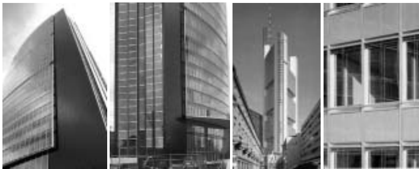
Figure 7.14 The ventilation inlets in the outer skin of the double façade of the ARAG Insurance company building make a rhythm of horizontal lines at every storey ( far left and left ). Double-height “sky-gardens” punctuate the building at every eighth floor. This is also accentuated in the façade with extra large ventilation inlets. The double façade of Commerzbank Headquarters is essentially made up of a single-glazed glass-layer located 0.15m in front of the openable windows in the inner skin of the facade ( right and far right ). There is an open slit in the outer glass-layer right under and right above each of the windows in the inner skin, which facilitates ventilation of the cavity. The outer glass layer dampens the pressure fluctuations created by wind, thus making it possible to apply openable windows in the inner skin.
