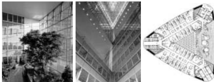
Figure 7.60 Sky-gardens ( left ) are connected with a central atrium ( middle ) in the Headquarters of Commerzbank (1997) in Frankfurt am Main. The inner perimeter of the v-shaped plan of offices ( right ) is ventilated towards the atrium/sky-garden, while the outer perimeter is ventilated through a double façade towards the outside.
