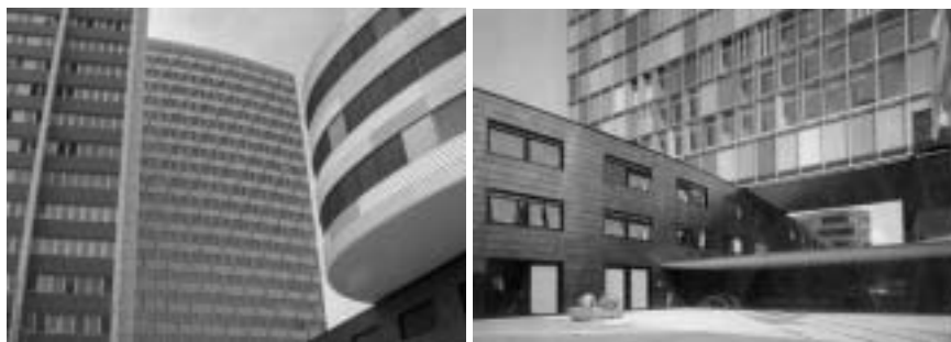
Figure 4.5 The picture (left) show (from left to right) the east façade of the existing tower, the high-rise and the Pillbox set atop the baguette. The high-rise building spans between the baguette and the baguettini (right).
