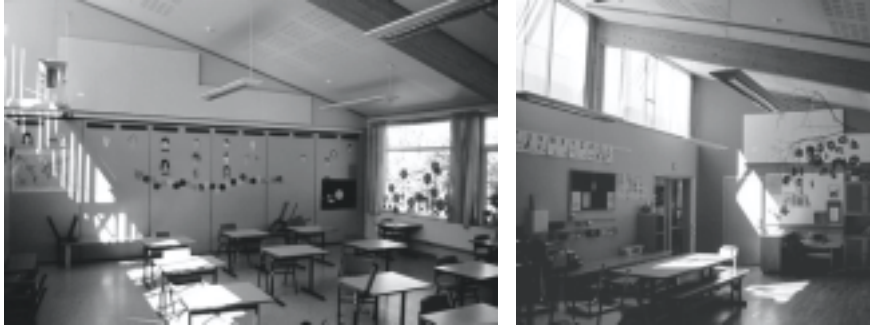
Figure 6.17 The sloping roof of the classrooms facilitate skylight in the core of the building.
