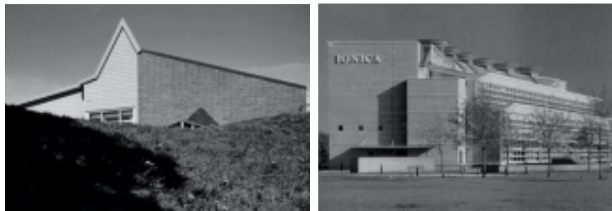
Figure 7.29 The roof of the Mediå Primary School (1998) in Grong, Norway ( left ) and the IONICA Headquarters (1994) in Cambridge, UK ( right ) both have an elevated central part in which ventilation air ascends before it is exhausted through wind tower(s). The shape of the roofs (and the gable wall in the Mediå case) are consequently characterised by an elevated ridge along the middle.
