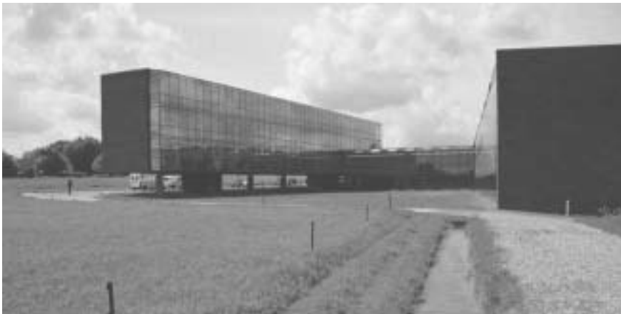
Figure 5.17 The U-shaped scheme opens up towards the meadows and the sea and turns its “back” to the car park.
