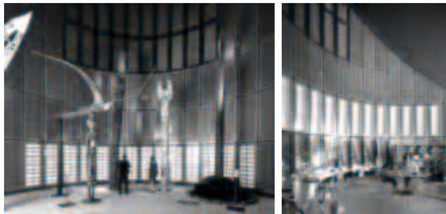
Figure 7.74 The interiors of the Jean Marie Cultural Centre in Nouméa, New Caledonia is characterised by the ventilation openings for inlets and outlets on the upper and lower part of the wall ( left ). The sloping roof reaches its highest point where the outlet openings are located ( right ).
