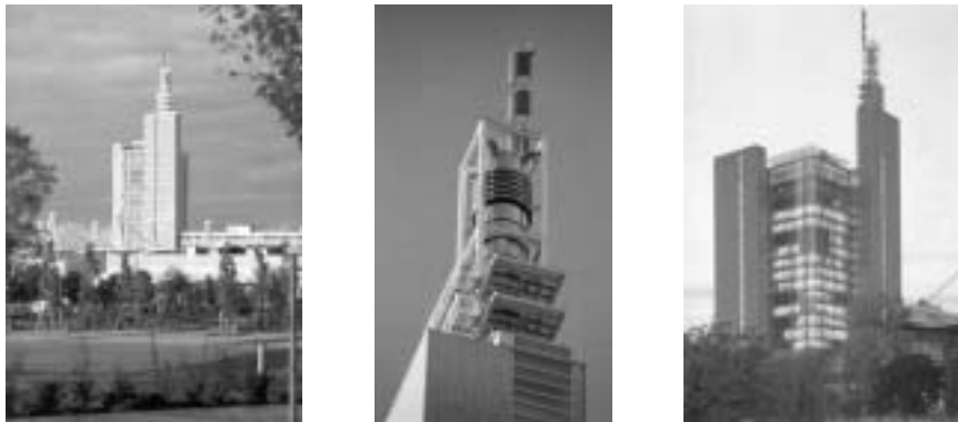
Figure 7.35 The exhaust chimney of the administration building of Deutsche Messe AG in Hanover, Germany distinguishes the silhouette of the building. (Passing by other points of comparison, the silhouette can be reminiscent of the statue of liberty in New York).
