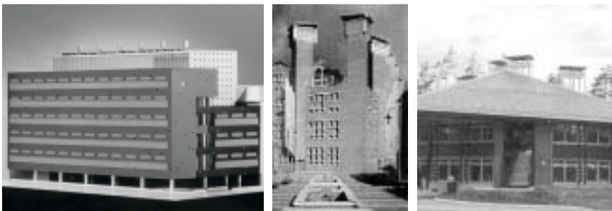
Figure 7.36 The silhouettes of the Tax Office in Enchede, Netherlands ( left ), the Lanchester Library in Coventry, UK ( middle ) and the Jaer School in Nesodden, Norway ( right ) are characterised by exhaust chimneys/towers for the natural ventilation. This is also the case for The Environmental Building in Garston, UK and the Inland Revenue Headquarters in Nottingham, UK (Figure 7.9).
