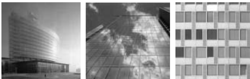
Figure 7.2 The Mitteldeutscher Rundfunk (MDR) Zentrale (2000) in Leipzig, Germany ( left ) has a double façade with horizontal ventilation openings on every storey. The administration building of the Deutsche Messe AG (1999) in Hanover, Germany ( middle ) has a double façade with a set of vertical ventilation openings located close to the corners of the building. The ventilation openings of the GSW Headquarters (1999) in Berlin, Germany ( right ) are scattered in a pattern onto the façade.
