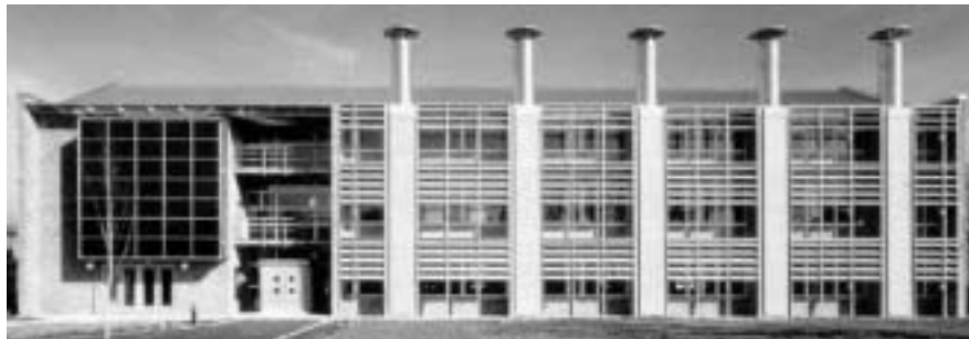
Figure 2.16 The BRE building with chimneys extending well above roof level to increase the stack potential and to achieve stable wind induced suction.
