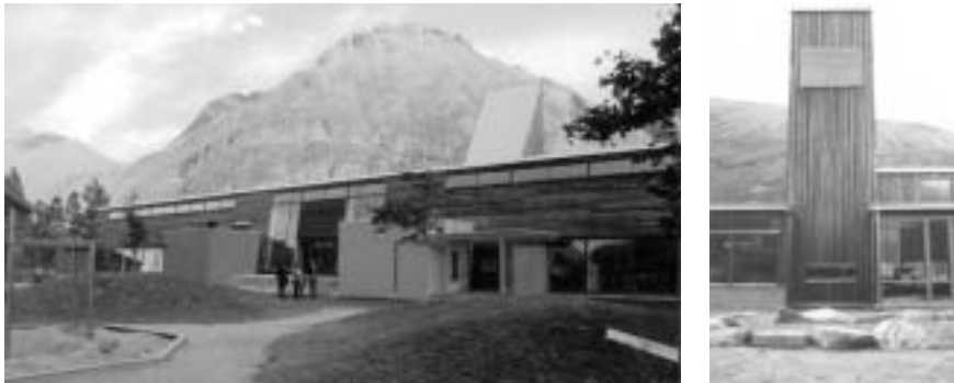
Figure 7.30 The exhaust tower of Tredal School in Sunndalsøra, Norway communicates with the surrounding mountain peaks ( left ), and introduces a strong vertical element in the otherwise rather horizontal building body ( right ).
