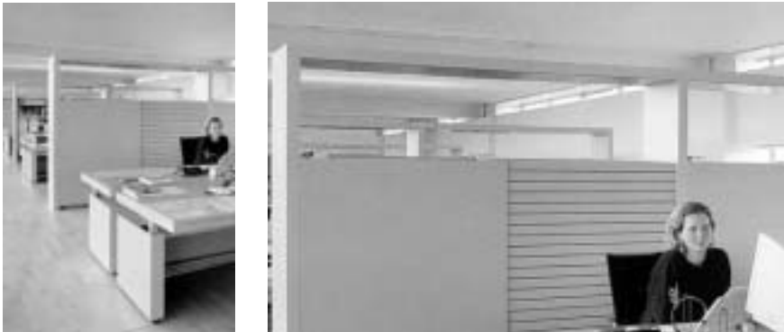
Figure 5.22 Acoustical attenuators are located in the bookshelf-walls behind each desk, appearing as a striped field in these walls ( left ). Note that the sliding mechanisms of the doors slide on top of the shelves, making it impossible to use the space on top for storage of paper, coffee cups and plants ( right ).
