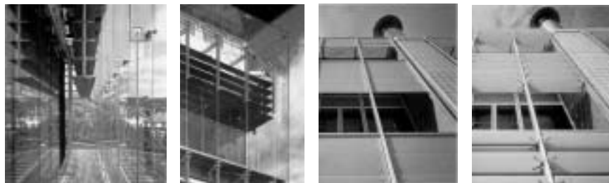
Figure 7.10 Two different manifestations of solar control illustrated by GlaxoWellcome House West Headquarters building (1995-97) in Greenford, UK ( far left and left ), and The Environmental Building of BRE (1994-96) in Garston, UK ( right and far right ). In the BRE building the translucent glass louvres in the bays span between the solar chimneys, and the rotating louvres are designed to cut out direct sun to the interior, whilst still letting in diffuse light.
