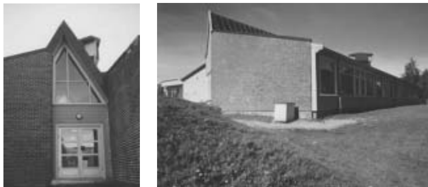
Figure 6.16 The east facing facade ( left ) and the north-east facing façade ( right ).
