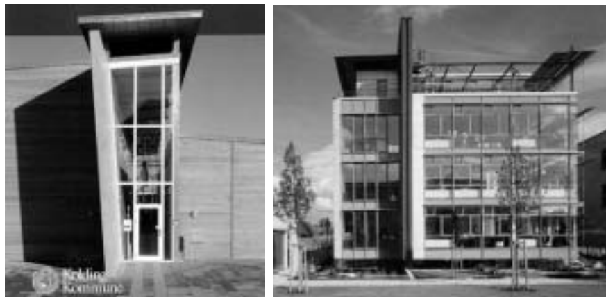
Figure 7.16 The central communication spine and exhaust stack of the Kvarterhuset (assembly building) in Kolding is “drawn out” and accentuated in the façade ( left ). The “black wall” (double solar wall used as extract for ventilation air) is accentuated in the east and west façades of the Headquarters building of Wasser- und Abfalltechnik Ingenieurgesellschaft (WAT) mbH in Karlsruhe ( right ).
