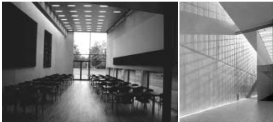
Figure 7.66 Acoustical attenuators are integrated in the artworks hung on the exposed concrete walls in the canteen of the Pihl & Søn Headquarters building in Lyngby, Denmark ( left ). The alignment of different materials with unlike texture and colour gives a sober impression and the materials accentuate each other. The in-situ cast concrete wall in the foyer of the B&O Headquarters building in Struer, Denmark looks, in combination with the skylight, almost like it is made of a “soft” textile-like material ( right ).
