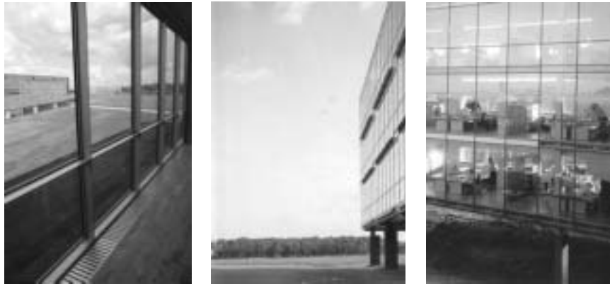
Figure 5.13 The inlet grills integrated in the floor next to the glazed north façade are made of aluminium and produced by B&O themselves ( left ). The manifestation of the inlet glass hatches in the north façade ( middle and right ).
