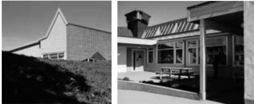
Figure 6.13 The extract chamber explains the “peak-shaped” ridge of the roof in the southern gable wall ( left ). The extract tower is located in the centre of the building where the two wings meet ( right ).
