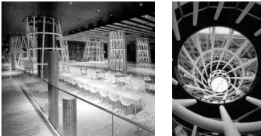
Figure 7.43 The reticular columns in the form of hyperbolic paraboloids penetrate the interiors as a struck of lightning. This analogy is not so far from “the truth” in that skylights set at the top of the columns transform them into “pillars of light”, feeding the interiors with daylight. The study of the form of the columns started out from the concept of a cylinder, subjected first to torsion and then deformed by oscillation. The torsion imparts greater stability to the structure. (Toyo Ito; works projects writings, 2002 ).
