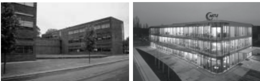
Figure 7.37 Together with the B&O Headquarters, the Pihl & Søn Headquarters in Lyngby, Denmark ( left ) and the building of DaimlerChrysler Aerospace, MTU Maintenance in Ludwigsfelde, Germany ( right ) are examples of buildings where the utilisation of natural ventilation does not affect the roof or the silhouette of the buildings.
