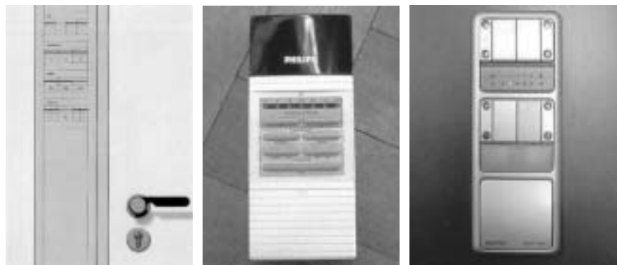
Figure 2.5 Panels in each office allow occupants a considerable degree of control over their particular environments in the RWE Headquarters in Essen, Germany ( left ). An infrared controller allows users to control lights and override the programmed settings of nearby windows and louvres in the Building Research Establishment’s (BRE) “Environmental Building” in Garston, UK ( middle ). Users can also open windows for local ventilation, and adjust roller blinds for additional glare control. An enhanced “light switch panel” provide the users with facilities for controlling lights, temperature, window openings and blind position in the Commerzbank Headquarters in Frankfurt-am-Main, Germany ( right ).
