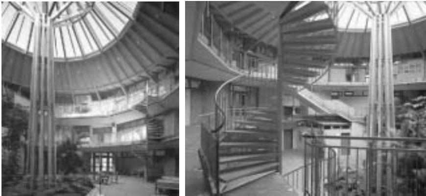
Figure 7.75 In addition to its social and visual functions, the central hall of the Waldorf School in Cologne, Germany serves as the main ventilation shaft. The stack effect is utilised to exhaust warm air through vents at the top and suck fresh air in at the bottom through inlets encompassed by greenery in the floor in the centre of the central hall ( left ). Galleries and stairs in the generously daylight central hall provide access to the classrooms and the different stories ( right ).
