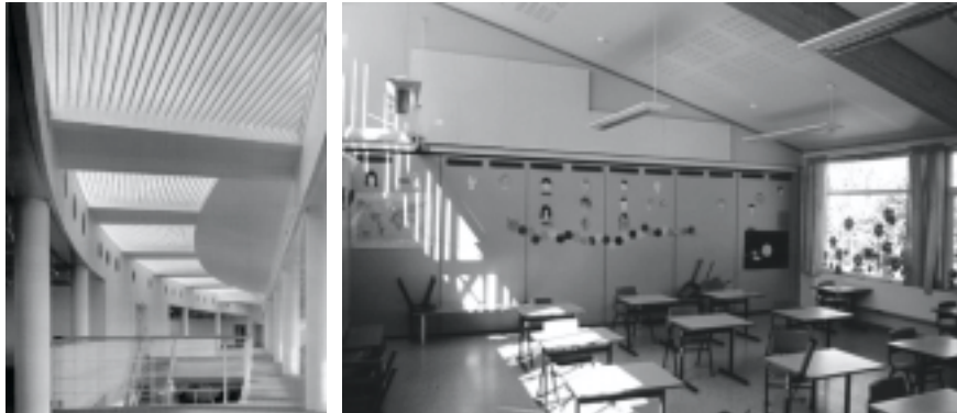
Figure 7.62 Both IONICA Headquarters in Cambridge, UK (left) and Mediå Primary School in Grong, Norway combine a centrally located extract of ventilation air with skylight windows that introduce daylight into the core of the buildings. (See also the Munkegård School in Figure 7.65, left ).
