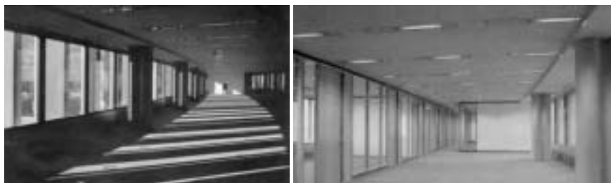
Figure 4.24 Pictures of an open plan layout ( left ) and a combi/west layout ( right ). The rhythm of slots in the ceiling containing lighting and technical installations can be seen in both pictures.
