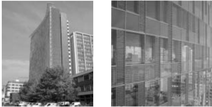
Figure 4.23 The west double façade and the wind roof are characteristic elements of the natural ventilation concept of the high-rise ( left ). The local ventilation inlets in the east façade also put a distinct mark on the building ( right ).
