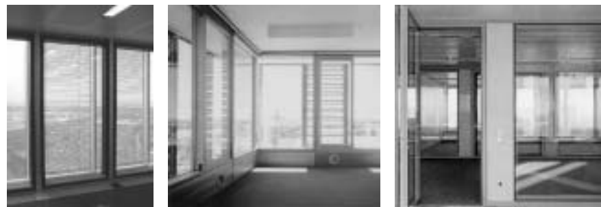
Figure 7.78 The pictures give an impression of how a double skin façade is perceived from the inside of the ARAG Headquarters in Düsseldorf, Germany ( left ), of the administration building of Deutsche Messe AG in Hanover, Germany ( middle ), and of the Commerzbank Headquarters in Frankfurt-am-Main, Germany ( right ).
