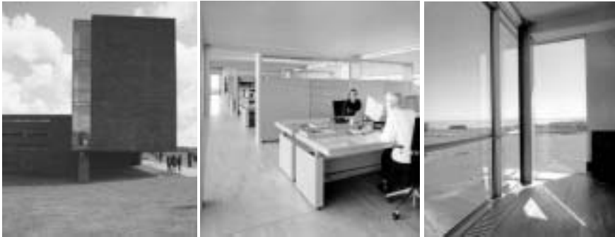
Figure 5.11 The gable façades of the office wing are identical (mirrored images of each other) and composed of a glass surface and a brick surface ( left ). The concrete is exposed both in walls and ceilings in the interior ( middle ). A view from the third floor towards Venø bay ( right ).
