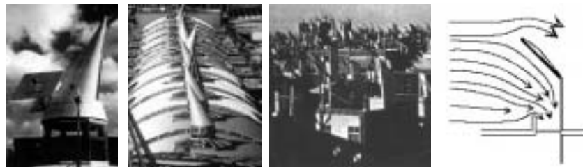
Figure 2.12 Full-scale mock-up of the wind scoop utilised in Blue Water Shopping Centre in Dartford, UK for performance monitoring ( far left ). The scoops are placed on the roof of the shopping mall with 15-metre intervals ( left ). Wind scoops in Dubai, United Arab Emirates ( right ) and a sketch of the wind scoop in principle ( far right ).
