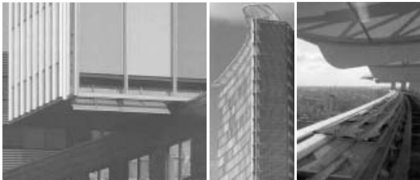
Figure 4.16 The air-path through the west double façade from the bottom opening ( left ), through the double façade (where exhaust air from every storey is collected) ( middle ) and finally at the top where exhaust air leaves the building under the wind roof ( right ).
