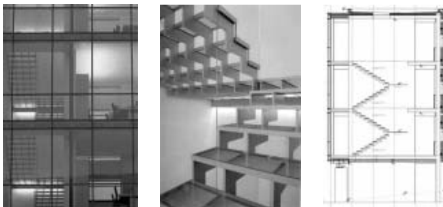
Figure 5.14 Two stairwells double as extract chimneys ( left ), and are designed to produce as little resistance for the airflow as possible ( middle ). They are centrally located in the plan with the outlet openings located immediately above ( right ).
