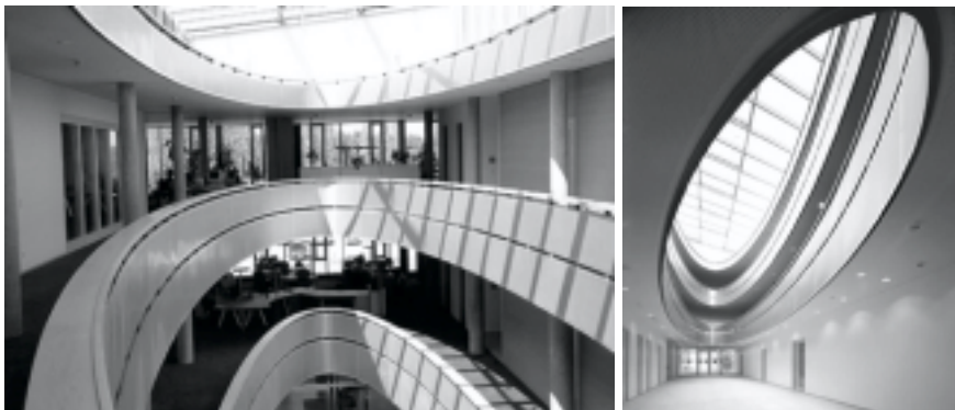
Figure 7.68 Flexible office spaces are organised around a central atrium in the DaimlerChrysler Aerospace building in Ludwigsfelde, Germany ( left ). The offices may be partitioned off and furnished as either clusters of office cubicles or large open-plan offices, team offices or flexible office landscapes. The atrium feeds the core of the building with daylight as well as serving as a stack chimney and extract air path for the building's natural ventilation concept ( right ).
