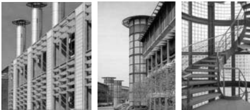
Figure 7.9 Solar chimneys in the façade of The Environmental Building of BRE (1994-96) in Garston, UK ( left ), and in the Inland Revenue Headquarters (1995) in Nottingham, UK ( middle ). The solar chimneys in the Inland Revenue buildings double as stairwells and are located at the corners of the building ( right ). The five solar chimneys of the BRE building are incorporated in the south façade. These chimneys are located in front of the actual façade, creating a row of bays.
