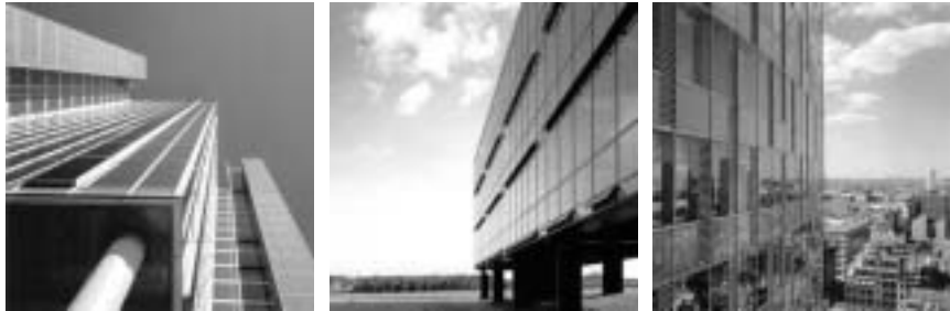
Figure 7.4 Pictures of three different buildings where the ventilation openings are located differently relative to the façade skin. The panels of the ventilation openings protrude from the façade of the administration building of Deutsche Messe AG (1999) in Hanover, Germany ( left ), whereas the glass hatches of the B&O Headquarters (1998) in Struer, Denmark open to allow airflow through ventilation openings set into the façade skin ( middle ). The panels of the ventilation openings in the GSW Headquarters are aligned with the façade skin ( right ).
