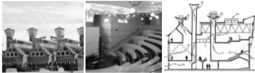
Figure 2.20 Skyline view of the naturally ventilated Queens Building, De Montfort University (1993) in Leicester, UK designed by Ford & Associates with Max Fordham & Partners ( left ). The auditorium in the building is also naturally ventilated ( middle ). The ventilation air enters through a large opening in the wall and is introduced to the supply chamber after passing through motorised volume-control dampers. From the supply chamber, it is distributed through voids under the seating and passes over finned heating tubes before being introduced in the atrium through a grille of aluminium mesh ( right ).
