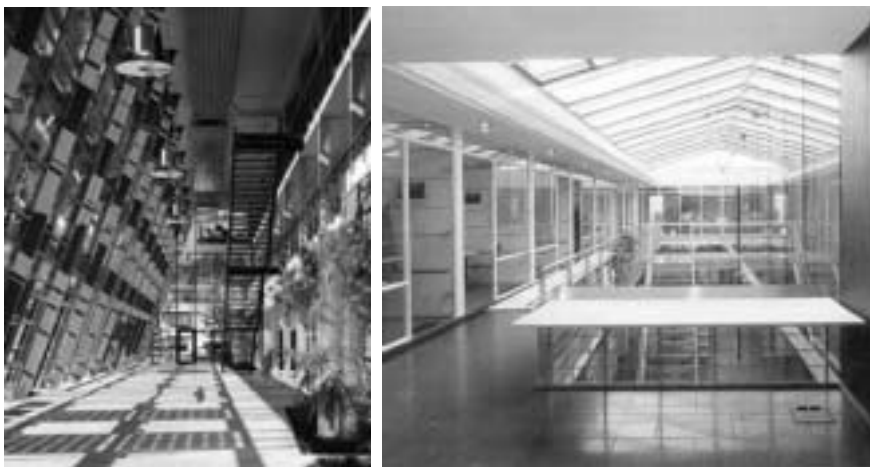
Figure 7.72 The linear shaped atrium of the Solar-Fabrik in Freiburg, Germany plays an important role in the natural ventilation concept of the building ( left ). The black glass-wall in the atrium of the WAT building in Karlsruhe, Germany serves as an installation wall and a ventilation chimney. Its stack effect is supported by the black colour which absorbs solar radiance ( right ). The atrium brings daylight into the core of the building and constitutes a central communication spine.
