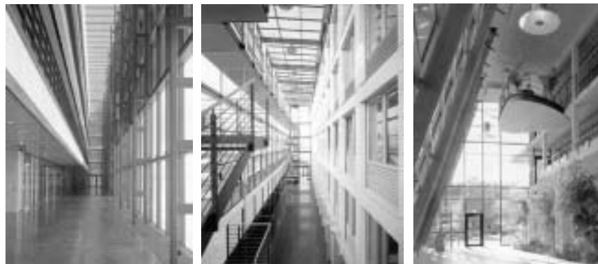
Figure 7.40 The atria/buffer zones of the develop centre of Audi AG (2000) in Ingolstadt ( left ), the Service centre of Nassauischen Sparkasse (2000) in Wiesbaden ( middle ) and the Solar-Fabrik Headquarters building (1999) in Freiburg ( right ) serve as vertical air paths and stacks for natural ventilation. They also house lobbies and vertical communication with stairs and galleries. (From the German Journal Intelligente Architektur ).
