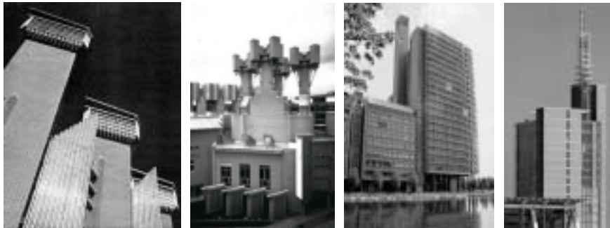
Figure 7.26 Four contemporary non-domestic buildings where chimneys are utilised in the natural ventilation concept. Lanchester Library and Learning Resource Centre at Coventry University (2000) in Coventry, UK ( far left ), The Contact Theatre (1999) in Manchester, UK ( left ), debis Haus at Potsdamer Platz (1996) in Berlin, Germany ( right ), and the administration building of Deutsche Messe AG (1999) in Hannover, Germany ( far right ). The two latter buildings show that natural ventilation has extended the use of chimneys to high-rise buildings. The design of the chimneys of the Lanchester Library and Learning Resource Centre and The Contact Theatre differ from the common conception of a chimney, as these chimneys are designed to react to changing wind and to allow rising air to exit without mechanical assistance under all weather conditions.
