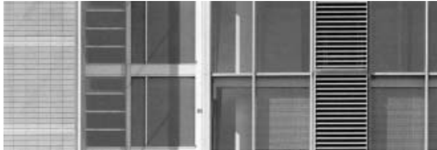
Figure 7.19 The grills in front of the ventilation inlets is a “new” element that contribute to enriching the façade of the administration building of Deutsche Messe AG in Hanover.
