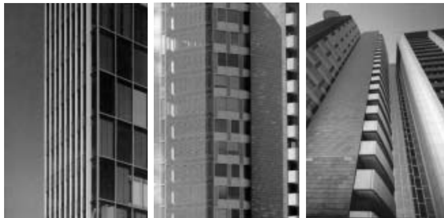
Figure 4.9 The north façade ( left ) and the south façade ( middle ) are both extremely narrow, accentuating the verticality of the high-rise. The meeting between old and new are exposed to the greatest extent in the south façade ( right ).
