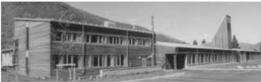
Figure 7.31 The direction of the weatherboarding in the east façade of Tredal School is used to underline the horizontality of the building and the verticality of the exhaust tower.
