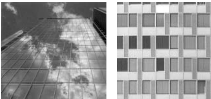
Figure 2.23 Vertical ventilation inlets located at the corners of the administration building of Deutsche Messe AG in Hanover, Germany ( left ) and a pattern of ventilation inlets in the east façade of the high-rise building of GSW Headquarters in Berlin, Germany ( right ).
