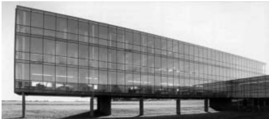
Figure 5.10 The glazed north façade of the elevated, rectangular shaped southern office wing.
